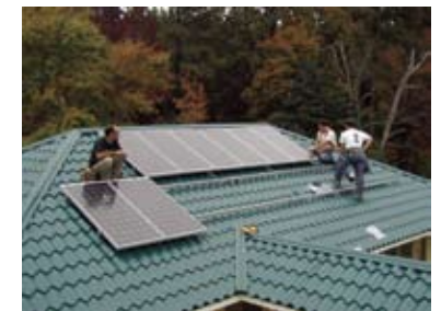
Builders installing photovoltaic solar electric system.
